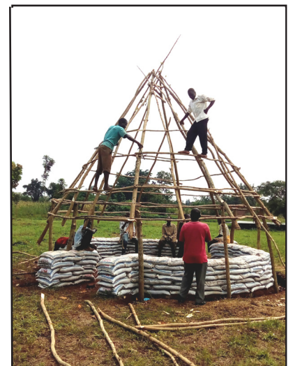
The meeting house being constructed
